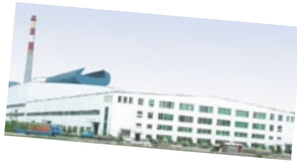
Overview of the entire Sichuan Malaya Glass plant in China.
